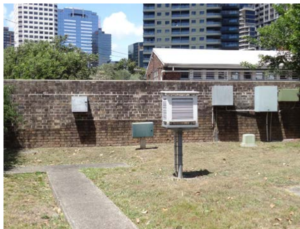
Figure 5. The small Stevenson screen in the cottage yard (27 December 2017) is dulled by road-grime. (The yard opens towards the Bradfield highway (left)). A 1966 photograph shows two screens on the camera-side of the 'T' at the end of the path separated from the school gymnasium (behind) by an open wire fence. Aerial photographs and data step-changes indicate the wall was probably built (or re-built) in 1972/73; sections affected by mortar-corrosion have been re-pointed. By trapping and radiating heat towards the screens and impeding airflow including cool-air drainage the wall changed the local heat balance.
